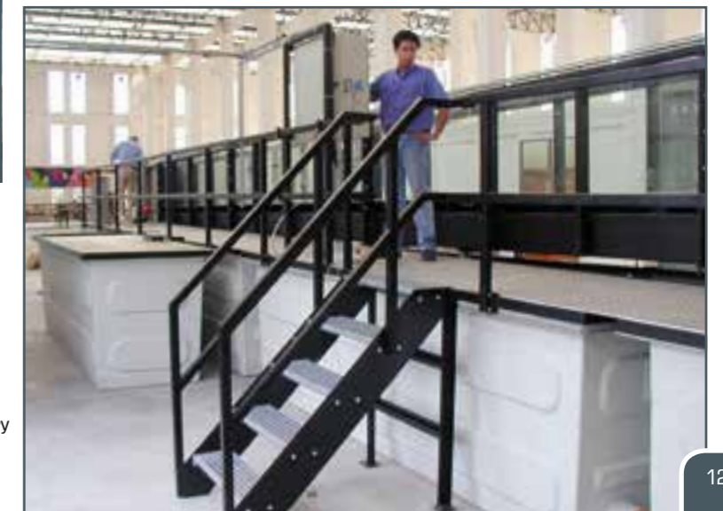
Element of the experimental section during on-site assembly. The elements are delivered ready for installation. Frames and beams are welded and painted. Tempered glass is used.
