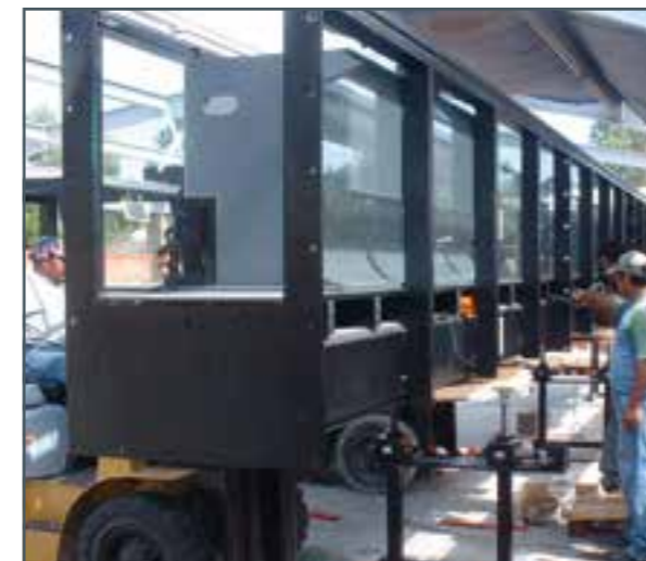
Element of the experimental section during on-site assembly. The elements are delivered ready for installation. Frames and beams are welded and painted. Tempered glass is used.
